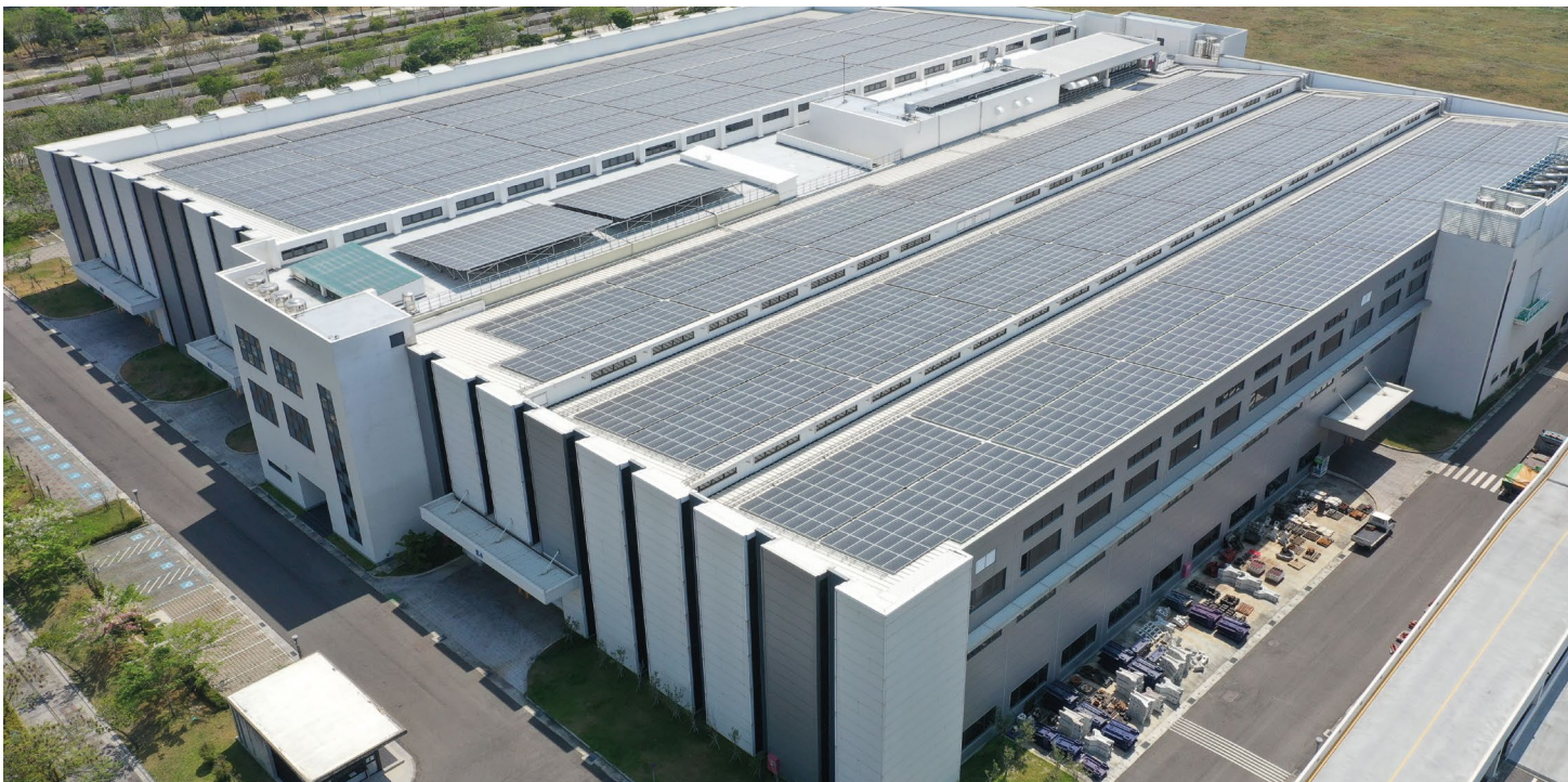
Insurers are cautious about covering property risks involving commercial flat roofs with solar PV installations
